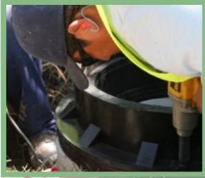
Manholes are often the first segment of a collection system to fail. Traditional concrete and metal systems are not designed to effectively handle their actual use — withstanding freeze-thaw cycles, heavy loads from traffic and a highly corrosive environment. When they inevitably crack and fail, water enters the collection system adding unanticipated flows. At the same time, the surrounding pavement is damaged.
