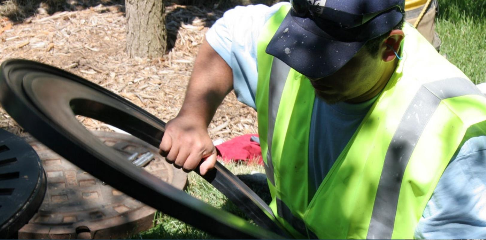
Integrated Frame and Adjustment Risers
